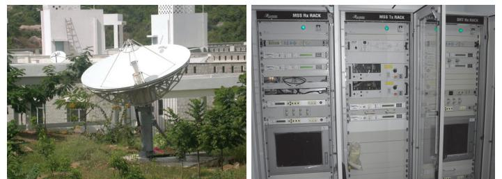
Communication facilities to receive data from seismic stations, tide gauges and BPRs in real time
