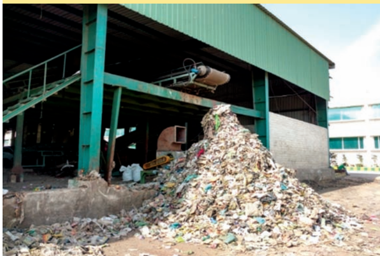
View of Ghazipur MSW landfill
